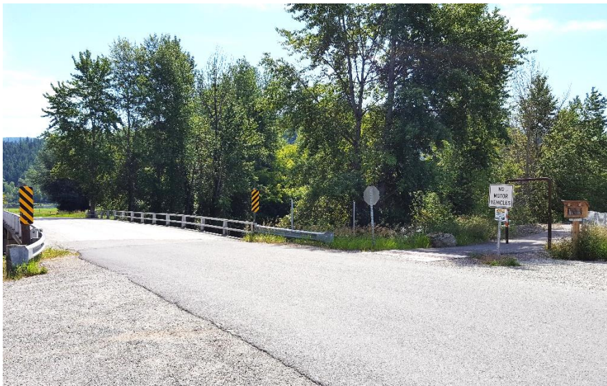
One of the entrances to J. Neils Trail from 5 th Street Extension.
