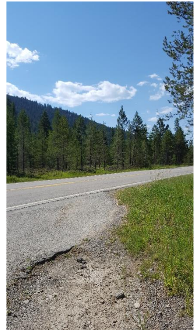
Crossing Pipe Creek Road
